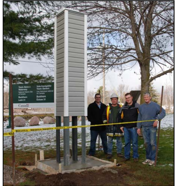
The tower at Lock 31 in Buckhorn immediately following installation.
