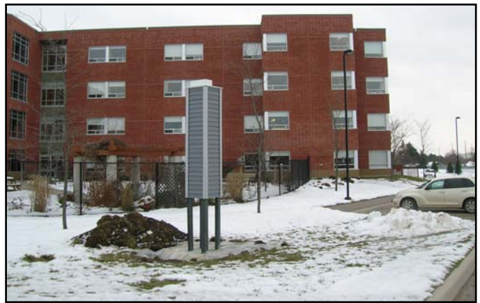
The tower at Fairhaven prior to the removal of concrete forms.
