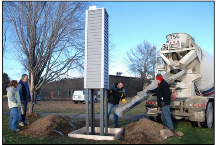
Installing the tower at Lock 20 adjacent to TSW offices.
