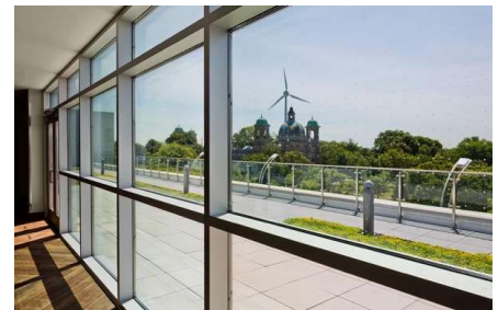
Example of AviProtek® bird-friendly glass with a discrete grid of white dots
